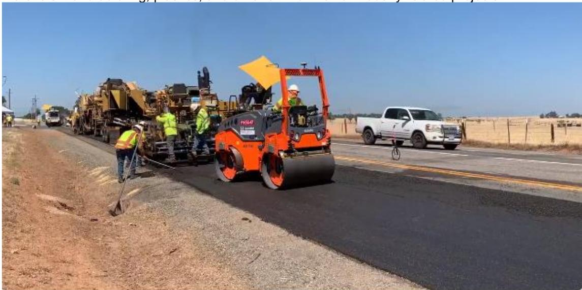
This may look like just an ordinary stretch of newly paved road, but it's being hailed as the first mile of recycled plastic highway on a state road anywhere in the U.S. Using more than 150,000 single-use plastic bottles, sustainable landscaping company [www.technisoil.com](http://www.technisoil.com) partnered with state transit officials to repave the one-mile stretch of three-lane road.
